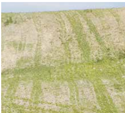
Rolling action after plant is very important
