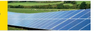
Fields need to be mowed in between the panel rows, as well as underneath and around panels. Without this upkeep, plants and grass can grow too high and shade or cover the panels, reducing their energy output.
